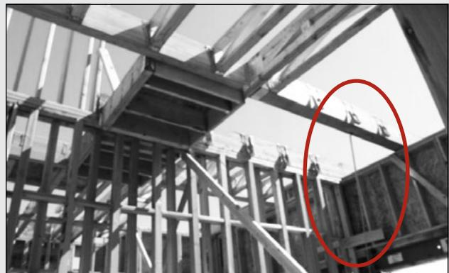
Photo of incident scene showing the opening the worker fell through while installing floor trusses
