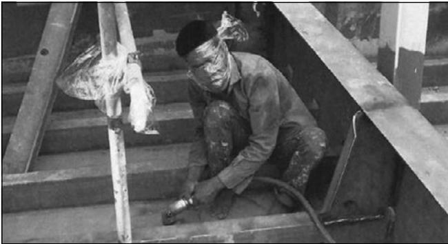
Assuming it doesn't suffocate him first, the makeshift Saran wrap face protection leaves the worker in this photo totally exposed to hazardous dust. What makes the picture especially irksome is that use of Saran wrap is an indication that somebody at the site recognized that the grinding work exposed the worker to respiratory hazards, yet nobody outfitted him with the proper respirator.
